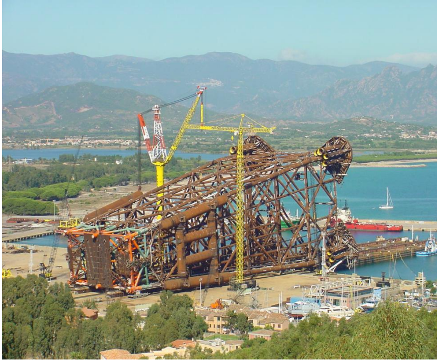
Sabratha Jacket Structure Weight 25,000 tonnes at Load out
