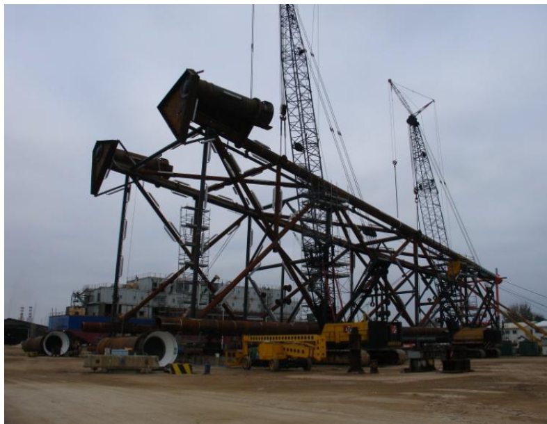
A small tripod Jacket Structure
