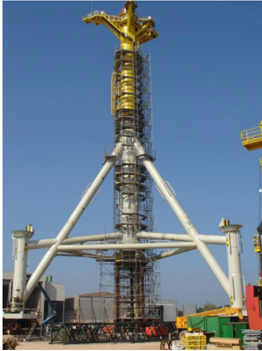
Monopod Jacket Structure - 71 meters high
