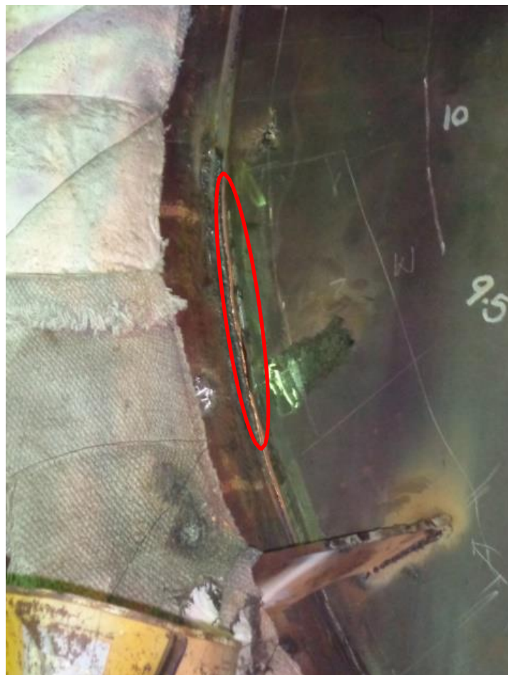
12B- Weld repaired to ensure proper root gap.
