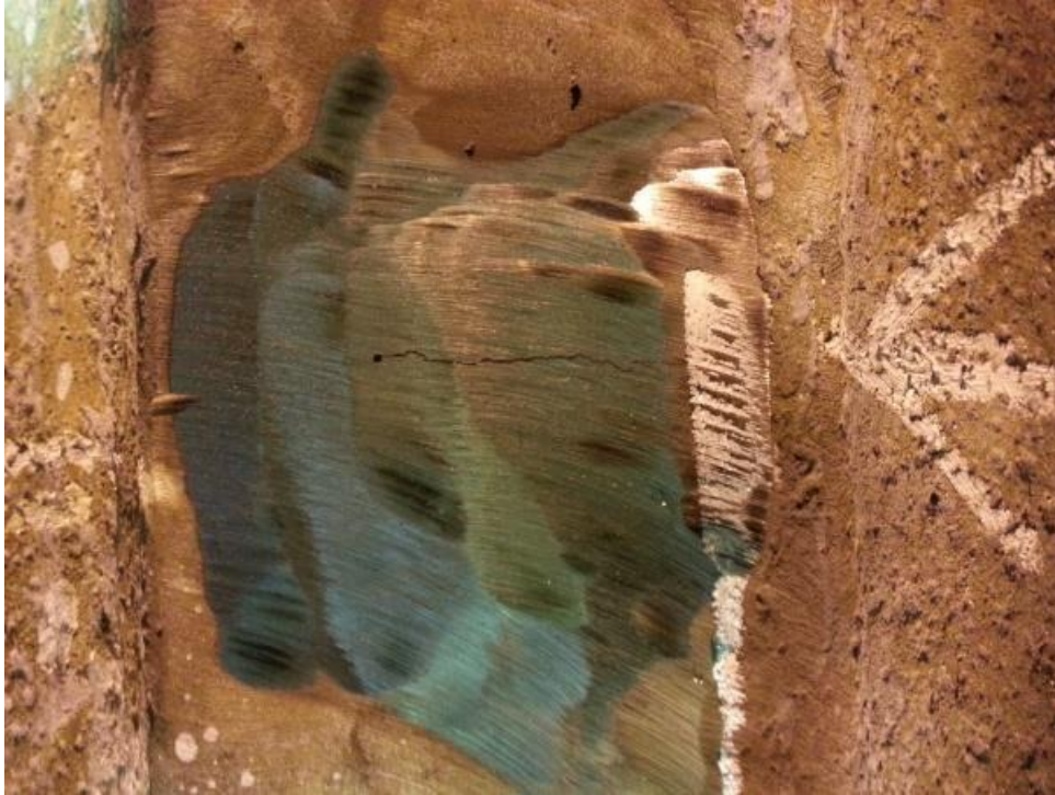
Fig.11B- Appearance of Transverse crack after grinding 8mm deep.
