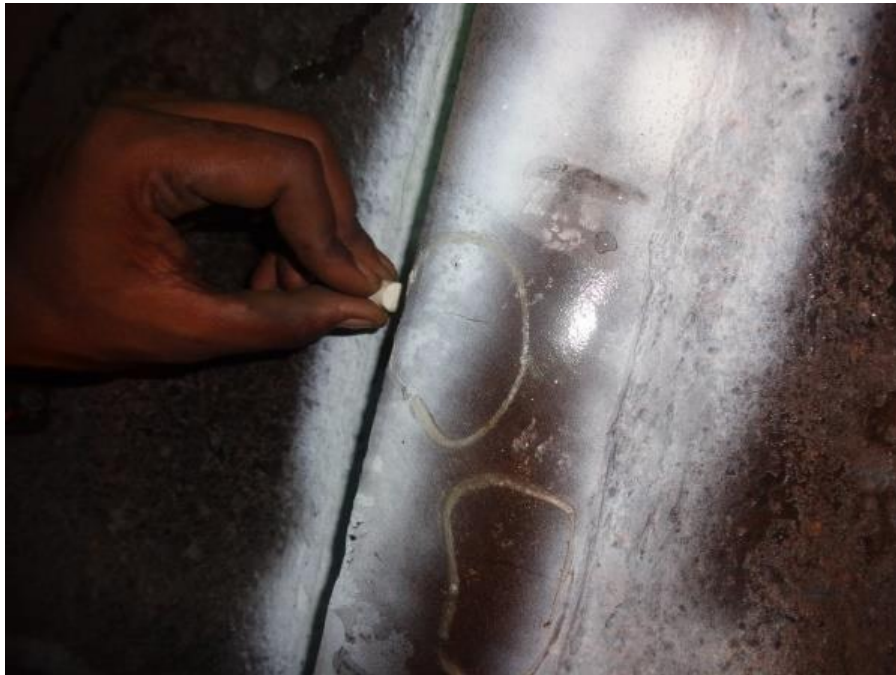
Fig.11A- Transverse cracks found during MT of Remaining Sickle Plate .
