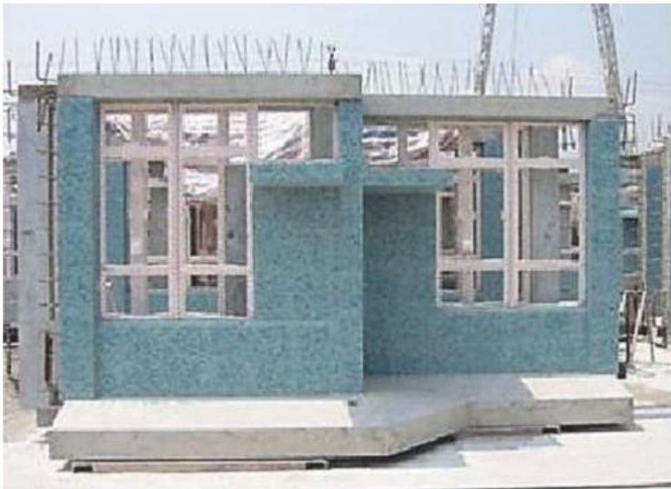
Fig. 33 Precast facade
