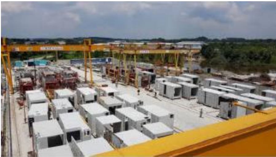
Fig. 68 Significant investment for factory to produce MiC modules
