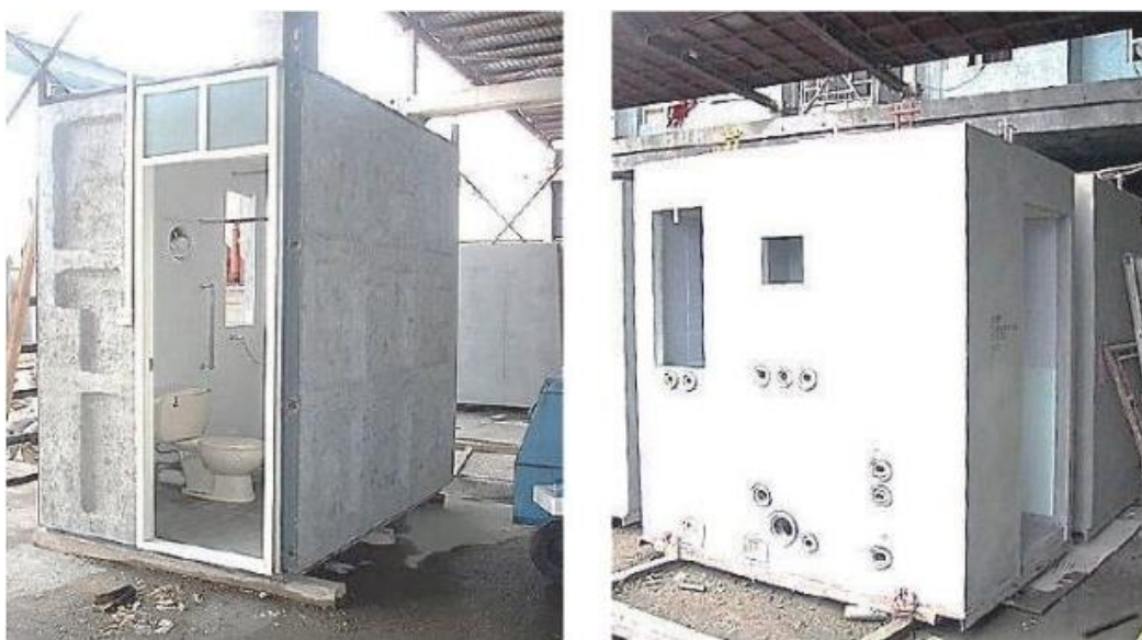
Fig. 49 Precast bathroom
