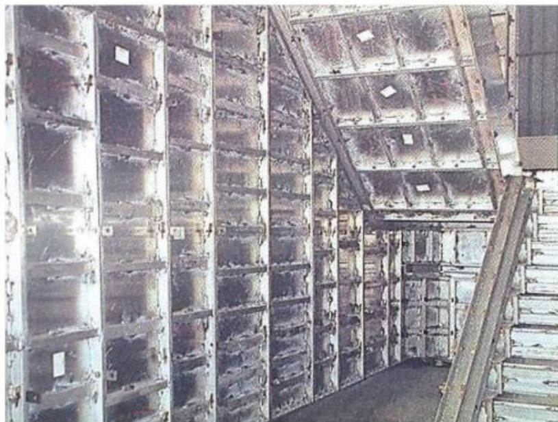
Fig. 54 Aluminum formwork
