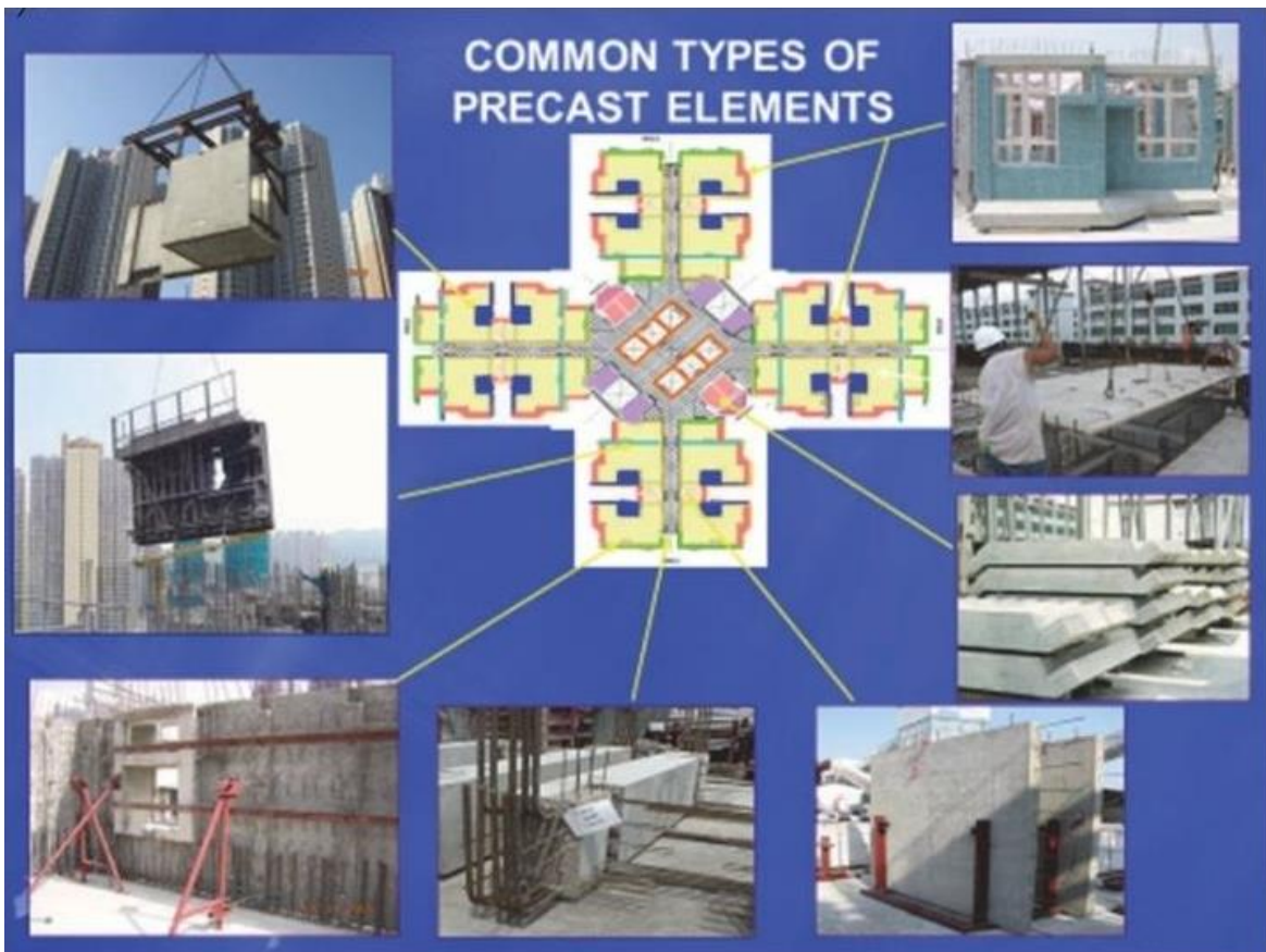
Fig. 29 Common types of precast elements
