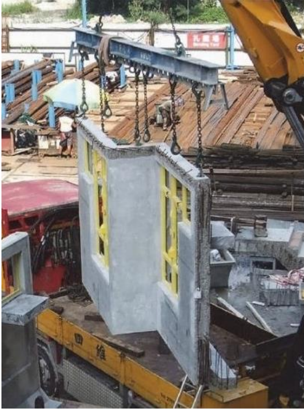
Fig. 37 Façade showing the lifting frame
