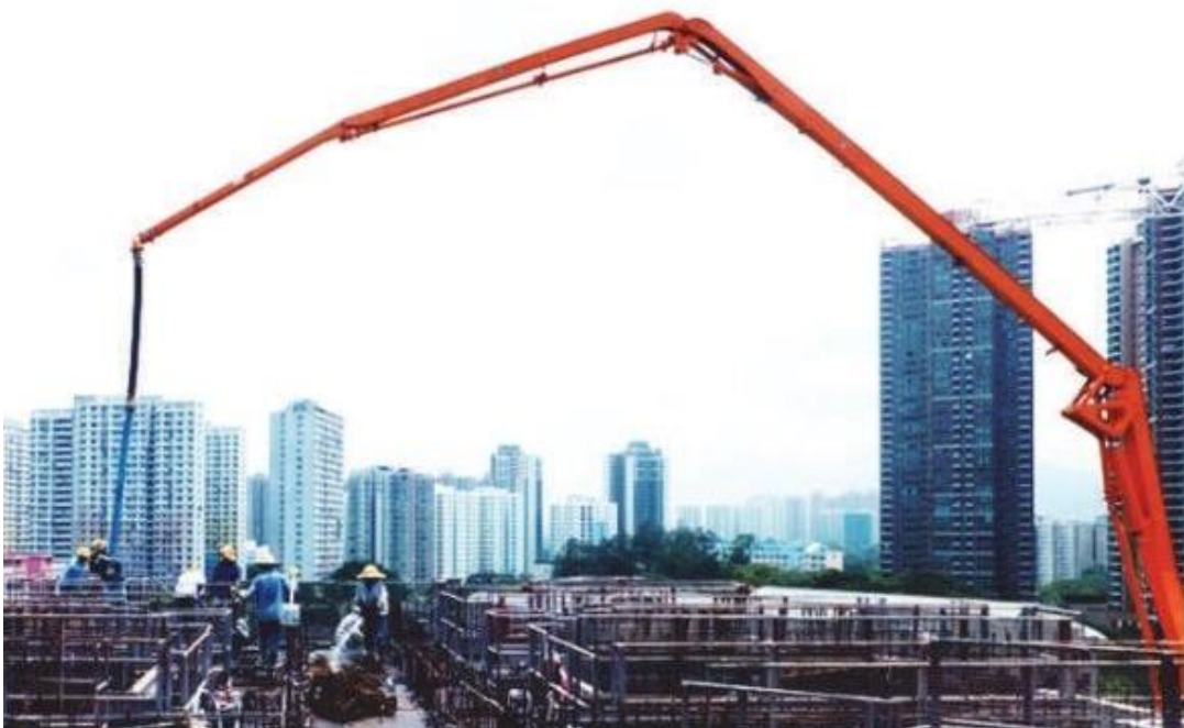
Fig. 63 Replacement of concrete skip with pumped concrete
