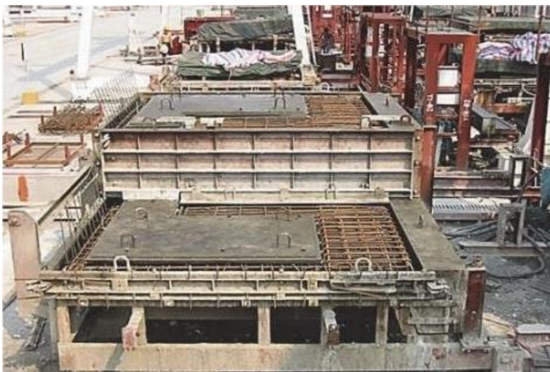
Fig. 32 Factory fabrication on ground
