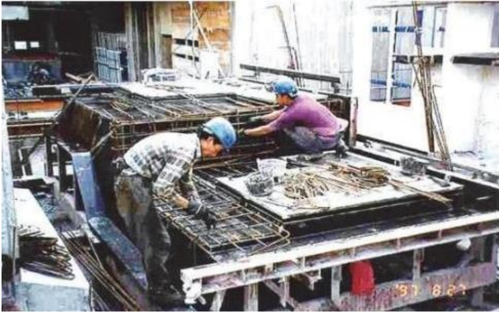
Fig. 34 Façade casting horizontally like a slab
