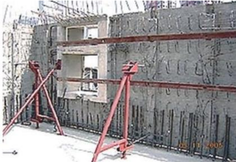
Fig. 48 Semi-precast wall
