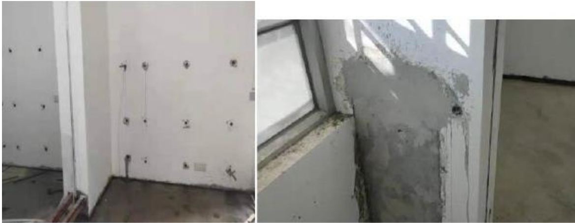
Fig. 75 Additional touch-up works
