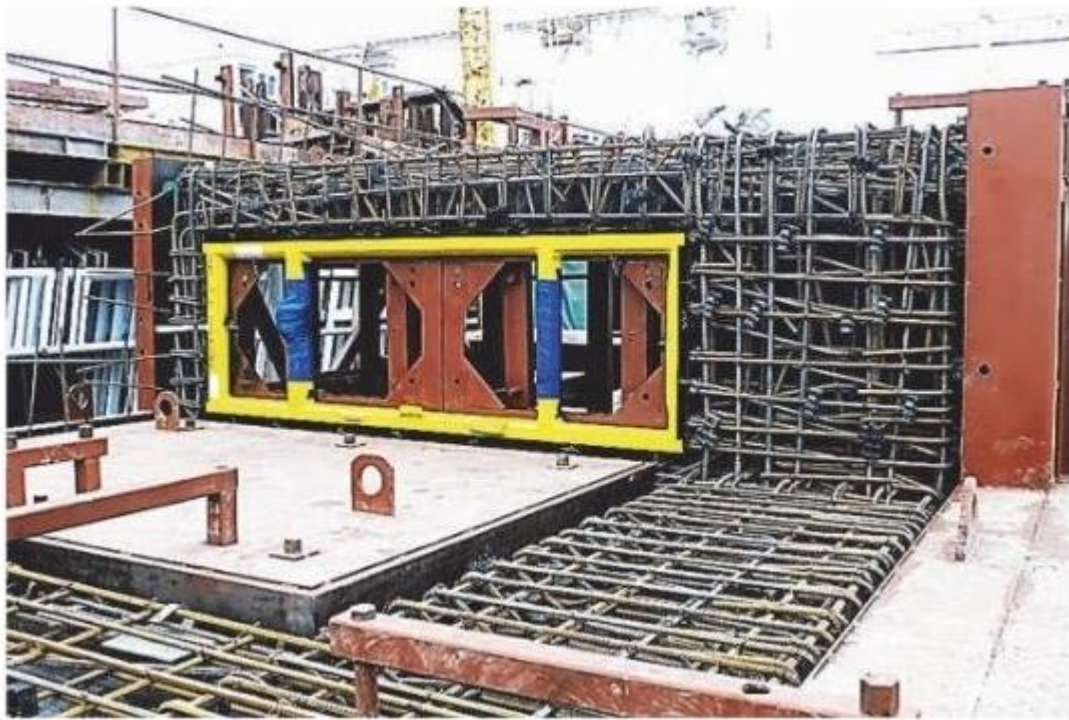
Fig. 66 Cast-in windows
