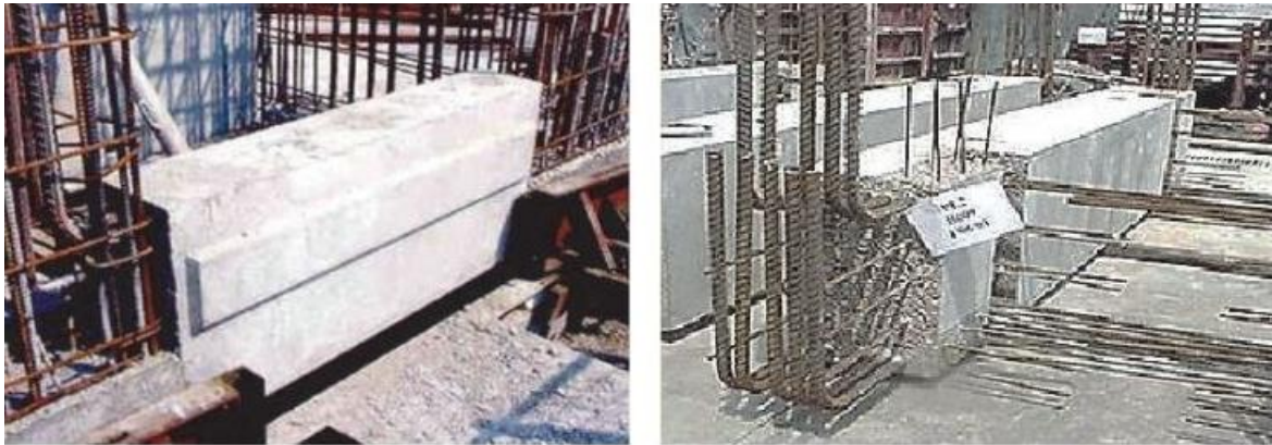
Fig. 47 Precast tie beam
