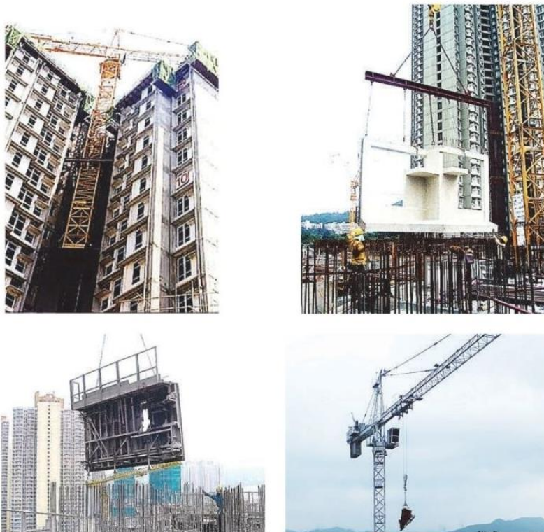
Fig. 62 Tower crane is heavily occupied
